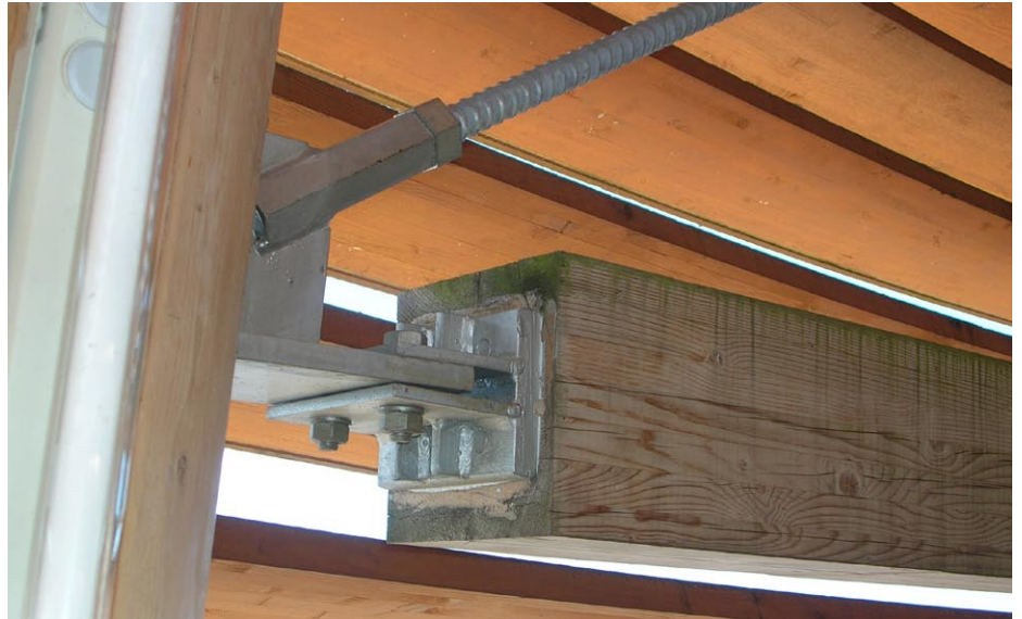
Bracing elements connected via steel brackets with Ferwood® anchored bolts.
