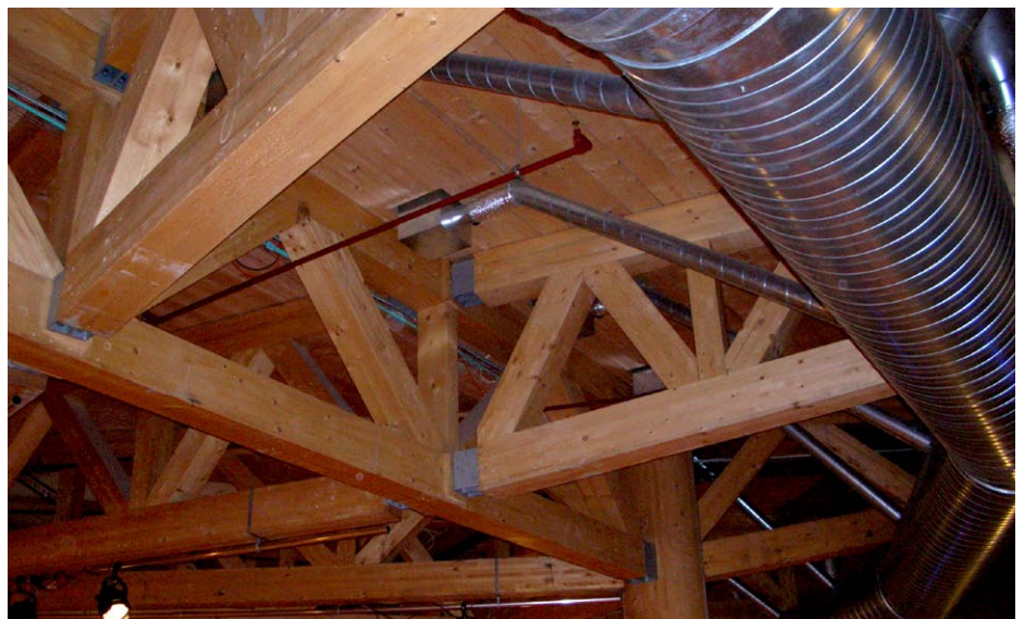
Structure supporting the first floor.
