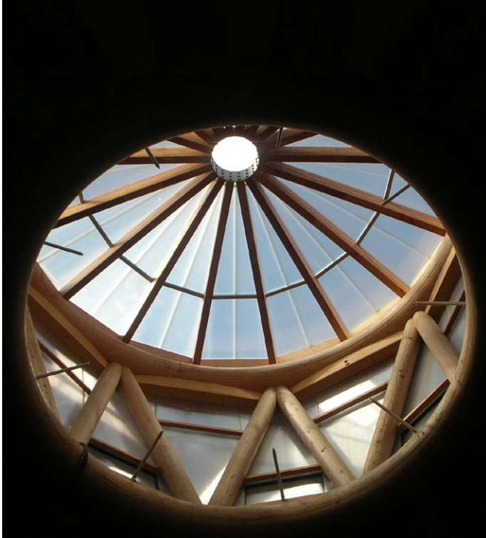
Central vortex and skylight.
