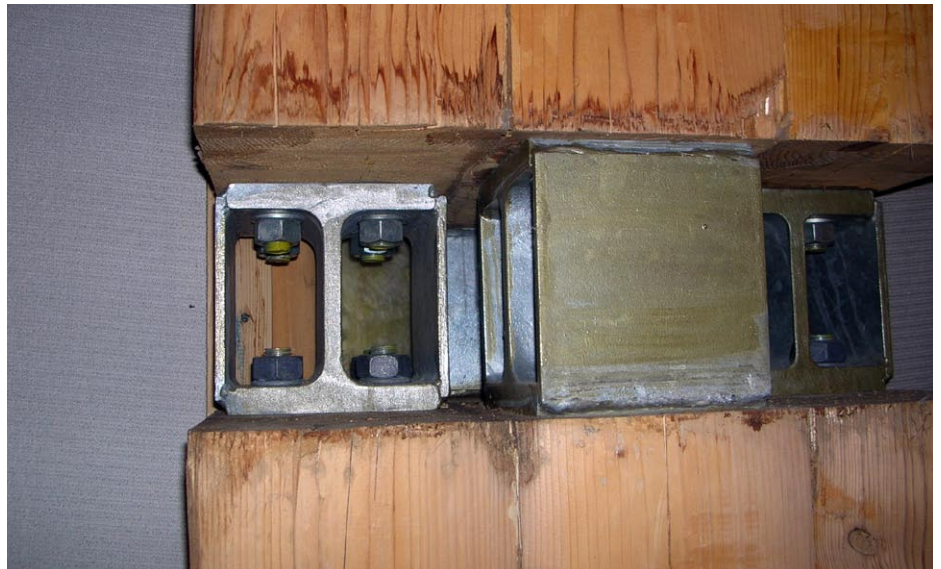
Steel sections with Ferwood® anchored bolts splice massive glulam arcs.
