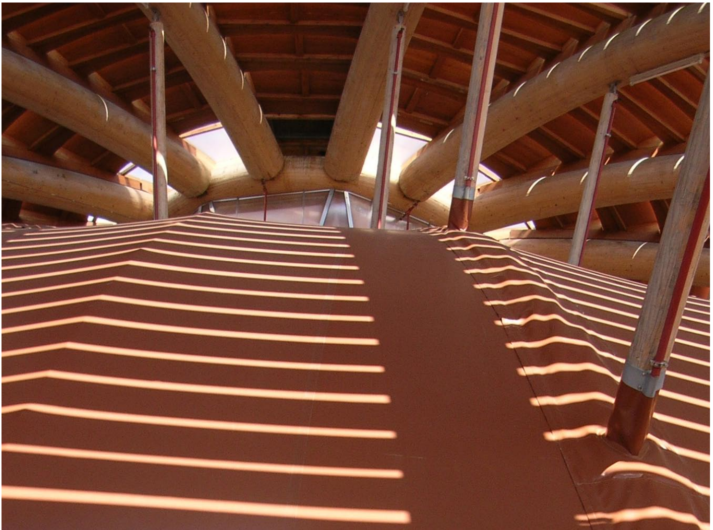
Weatherproof membrane over inner shell.
